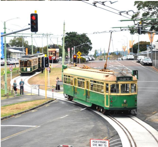
Rail laying and grinding
